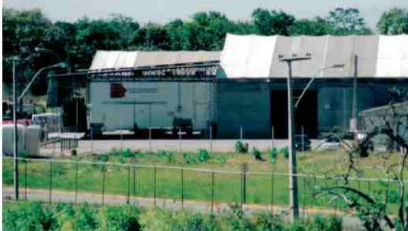
The Ceará state investment in cold storage facilities for flowers at the airport has assumed a major character in export logistics.
